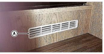
Fig.6.1 - Permanent ventilation openings
